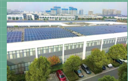
Introduced solar power generation at all production plants
