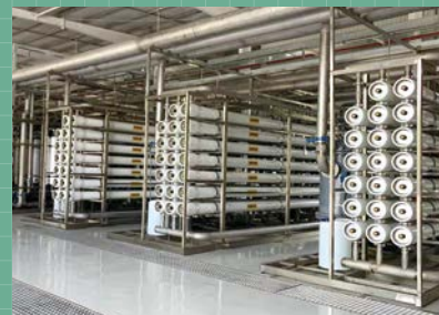
Reverse osmosis (RO) water treatment system for reusing water
