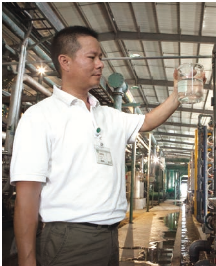
Frequent checks for appropriate effluent disposal
